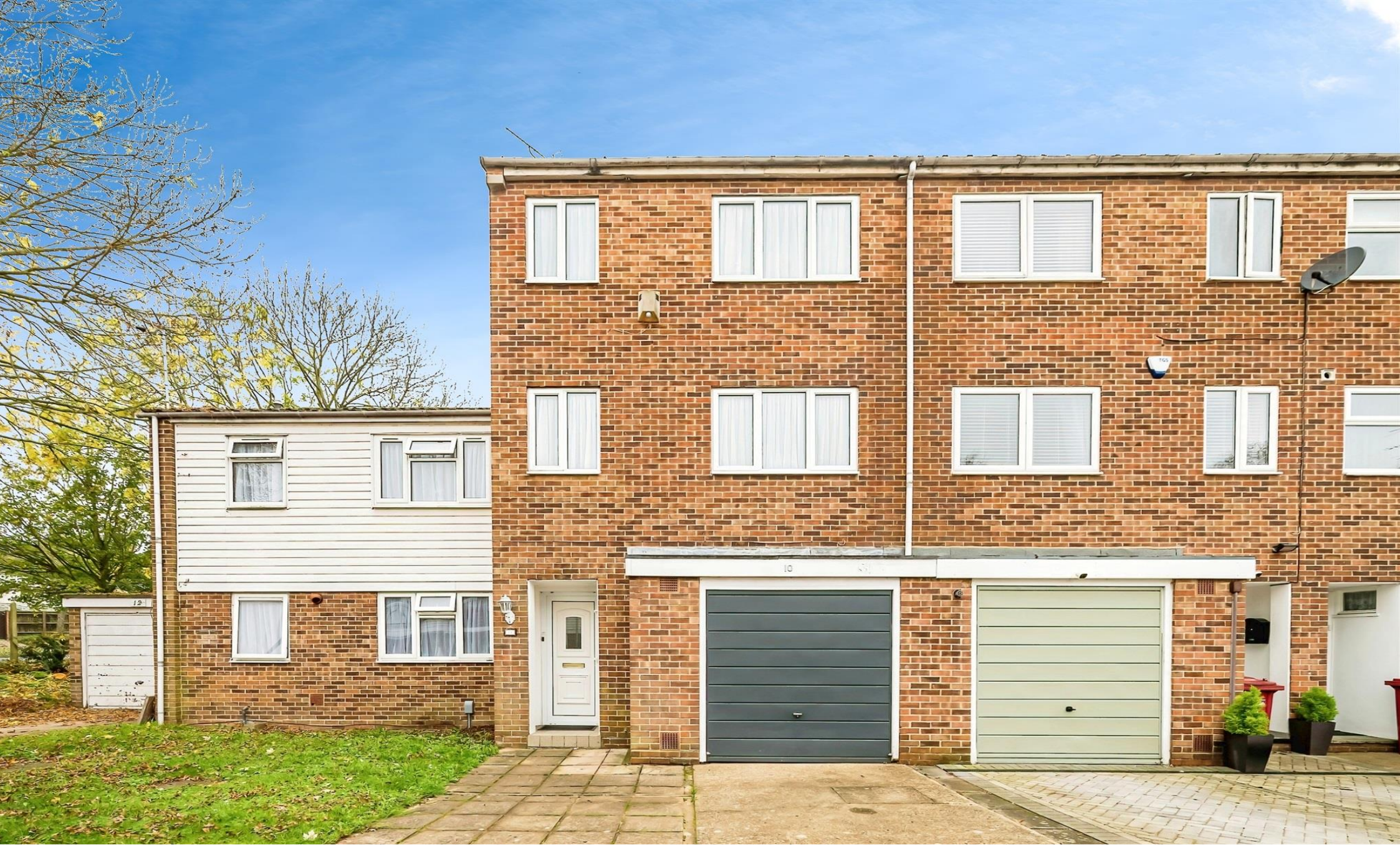
Tennyson Way, Slough SL2 2PA
