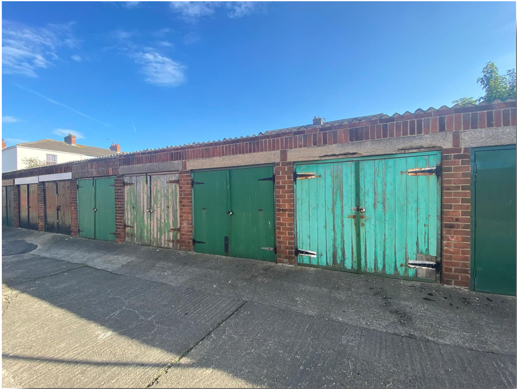
Garage East View Terrace, Hartlepool TS25 1AN
