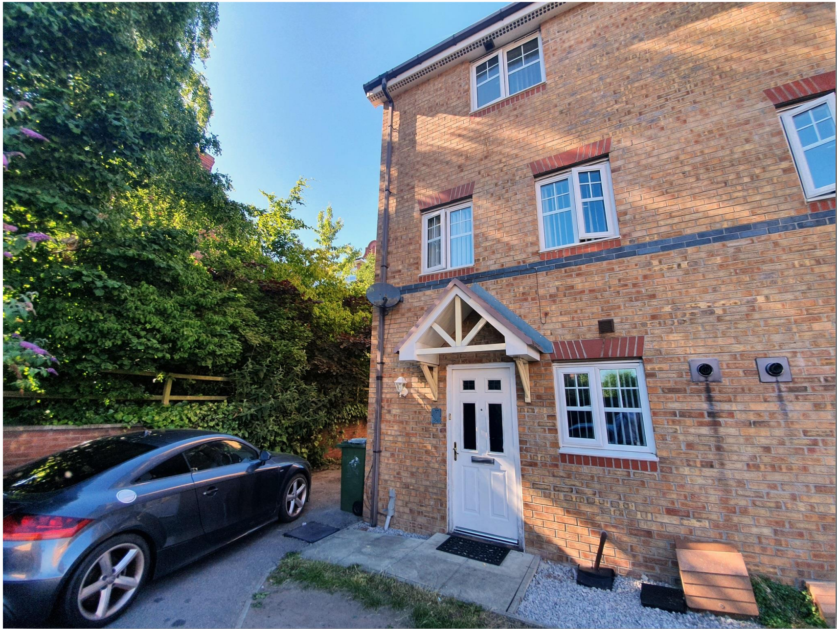
Merlin Road, Birkenhead, CH42 9QG
