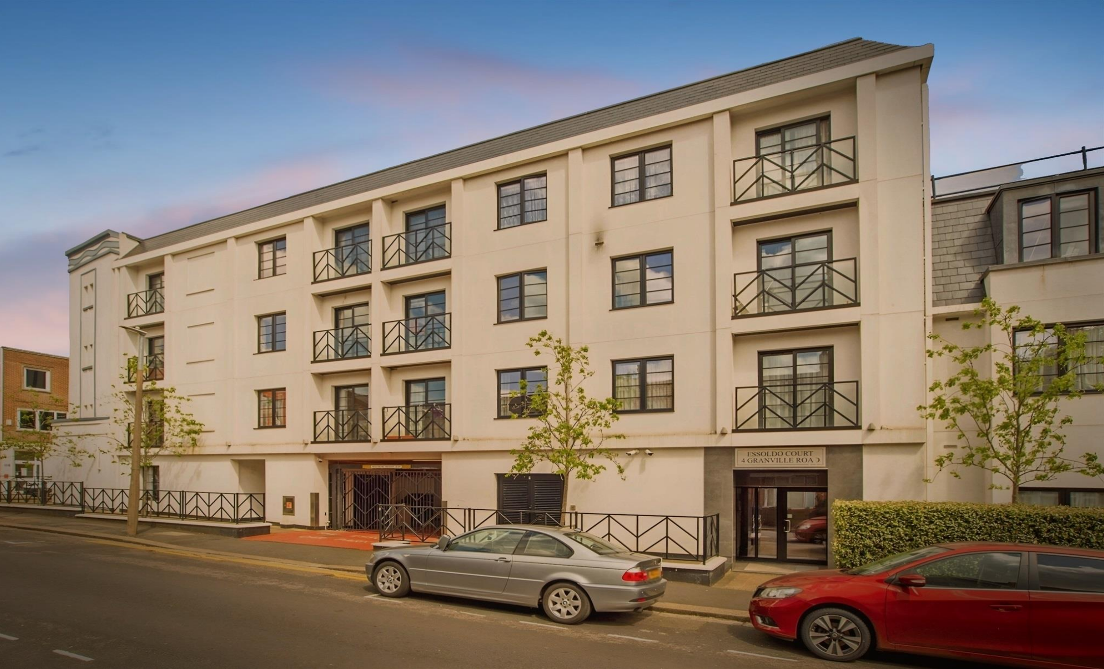
Essoldo Court Granville Road Watford
