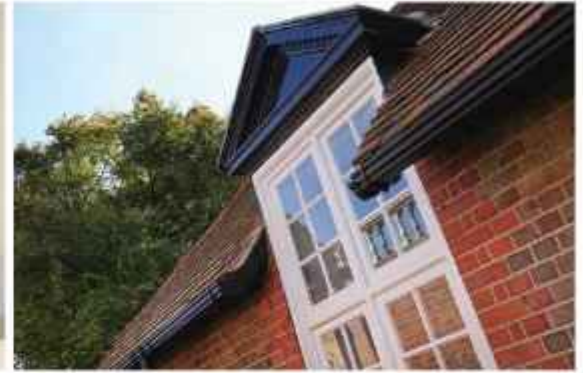
New or newly renovated single glazed timber windows
