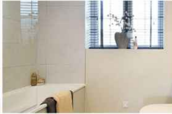
Ceramic wall tiling in bathrooms, shower rooms and en-suites
