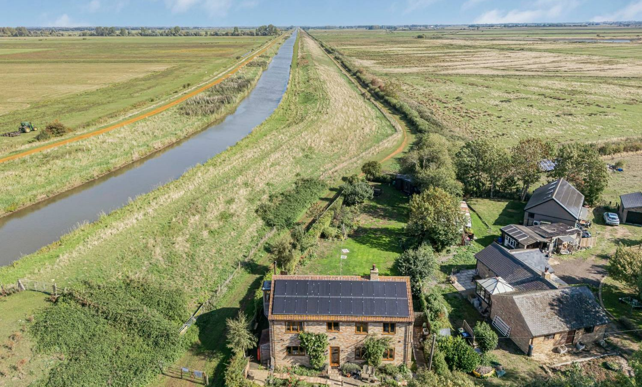
River Toll Cottage Hive Road, Witcham Ely
