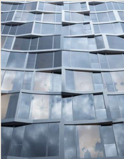
DOUBLE GLAZED INSULATED LOW-E FAÇADE
