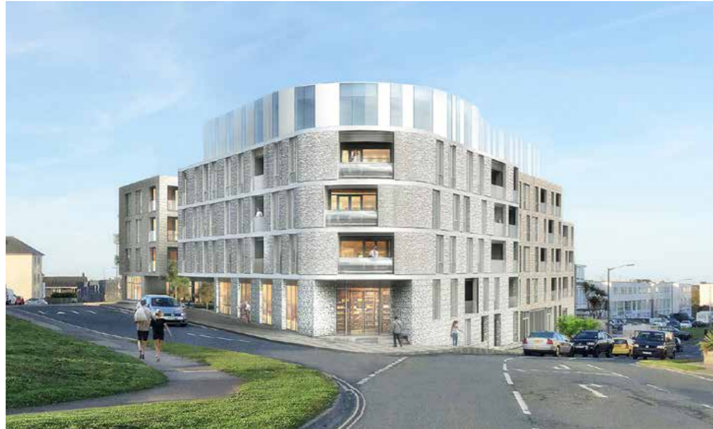
CGI of One Pentire as seen from Pentire Road.
