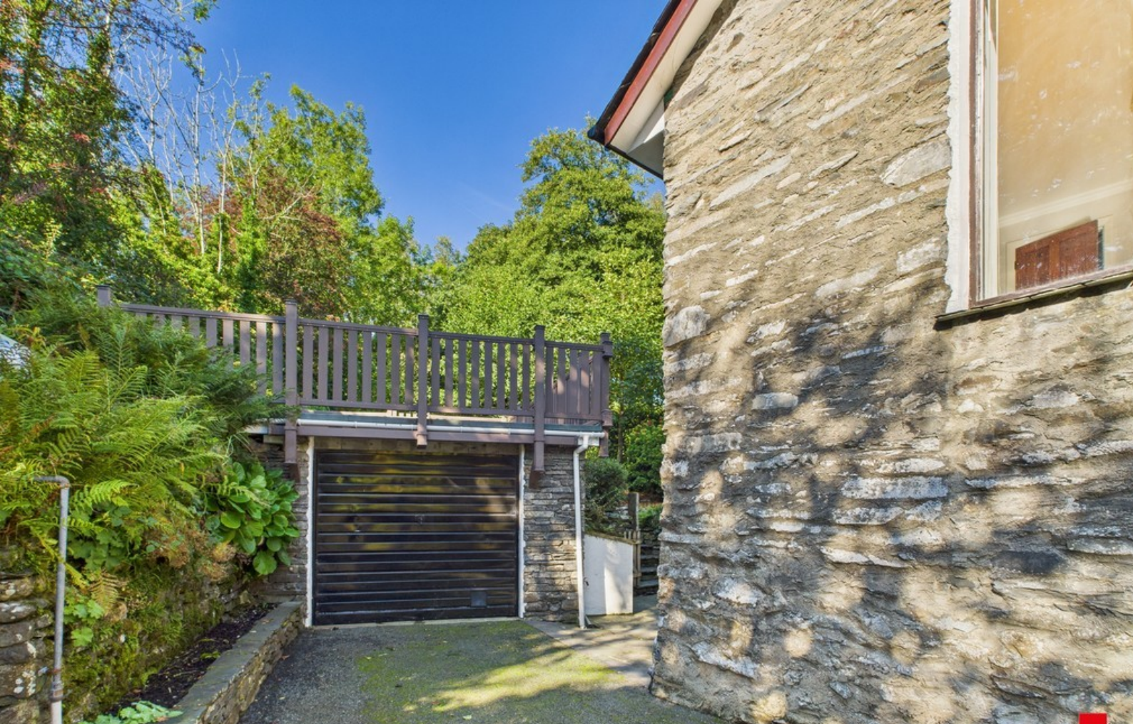
Detached Garage/Workshop Patio Area above
