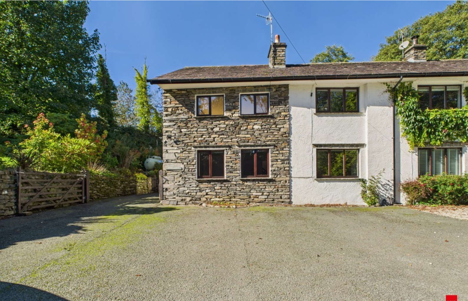
External and Parking Area
