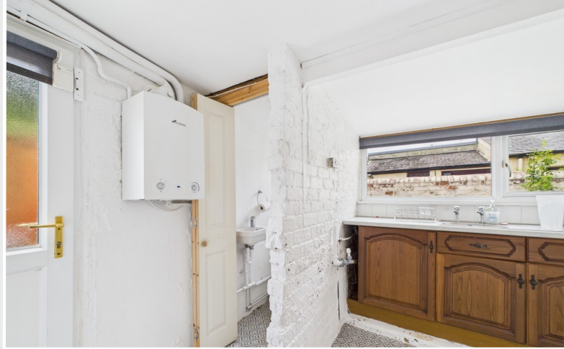
Utility and WC
