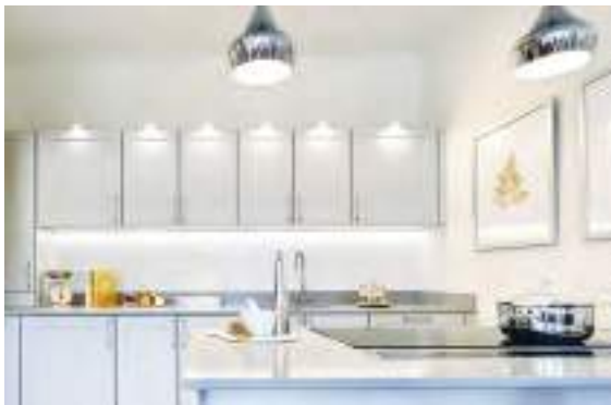
Low energy pendant lights and LED downlights
