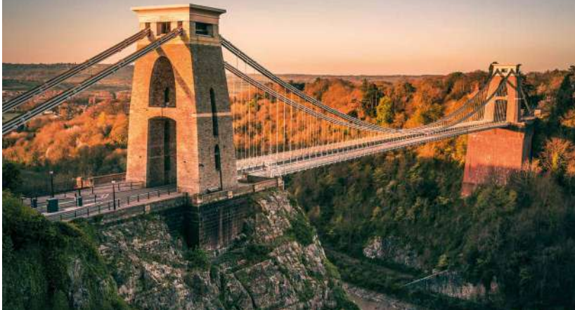
Clifton Suspension Bridge in nearby Bristol.
