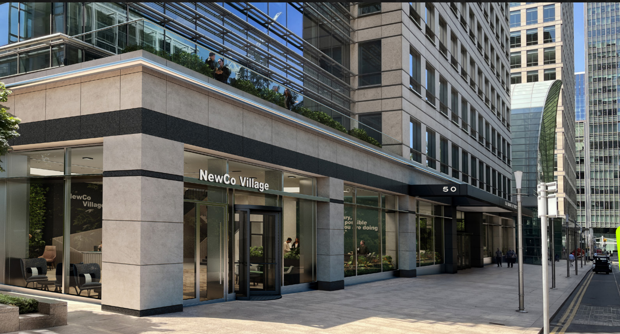
Self-contained entrance exterior CGI
