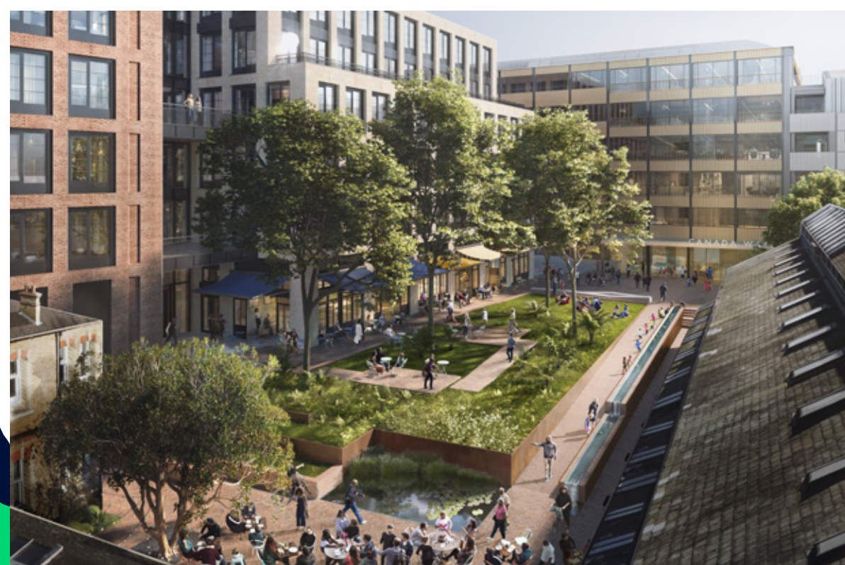
Dock Office Courtyard PC late 2024
