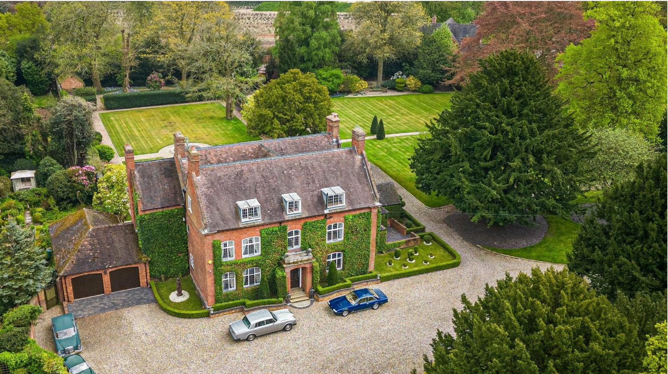
Wall House, Green Lane, Wall
