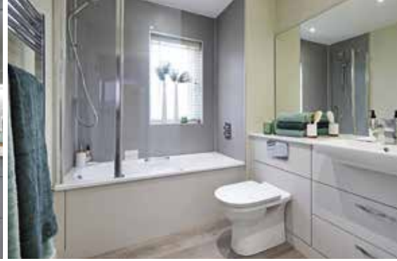
Easy-to-clean bathroom wall panelling provides a hygienic alternative to tiling and grout
