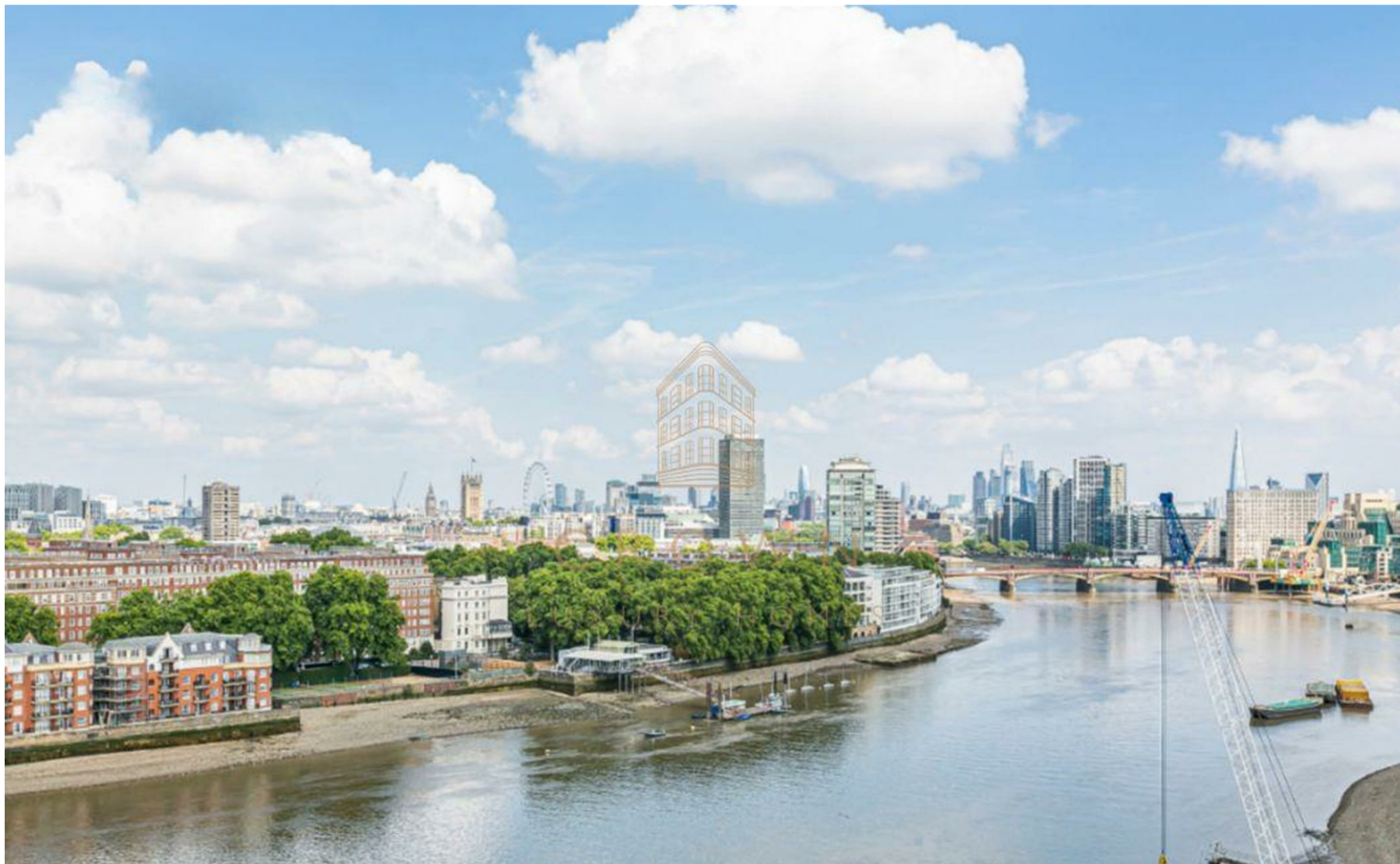
Apartment 200b, 3 Riverlight Quay, London, SW11 8BF £6,500
