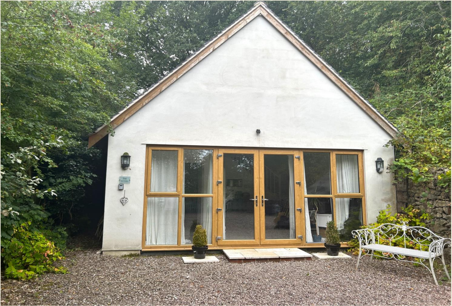
DETACHED TWO STOREY ANNEXE:-
