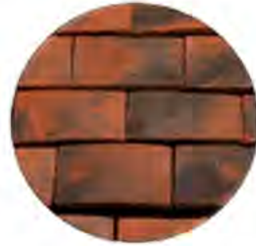
Clay Tiled Roofing
