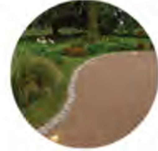
Permeable Resin Bound Gravel
