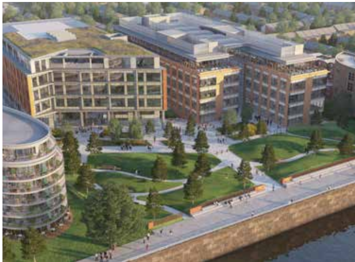
The Refinery, Mambre Wharf
