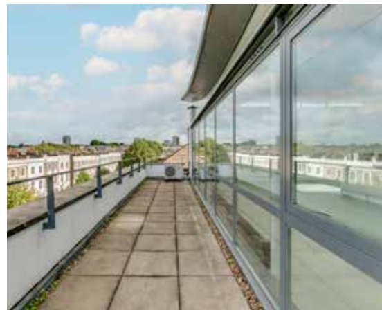
4th floor terrace
