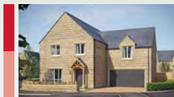
The Prestleigh 5 BED DETACHED
