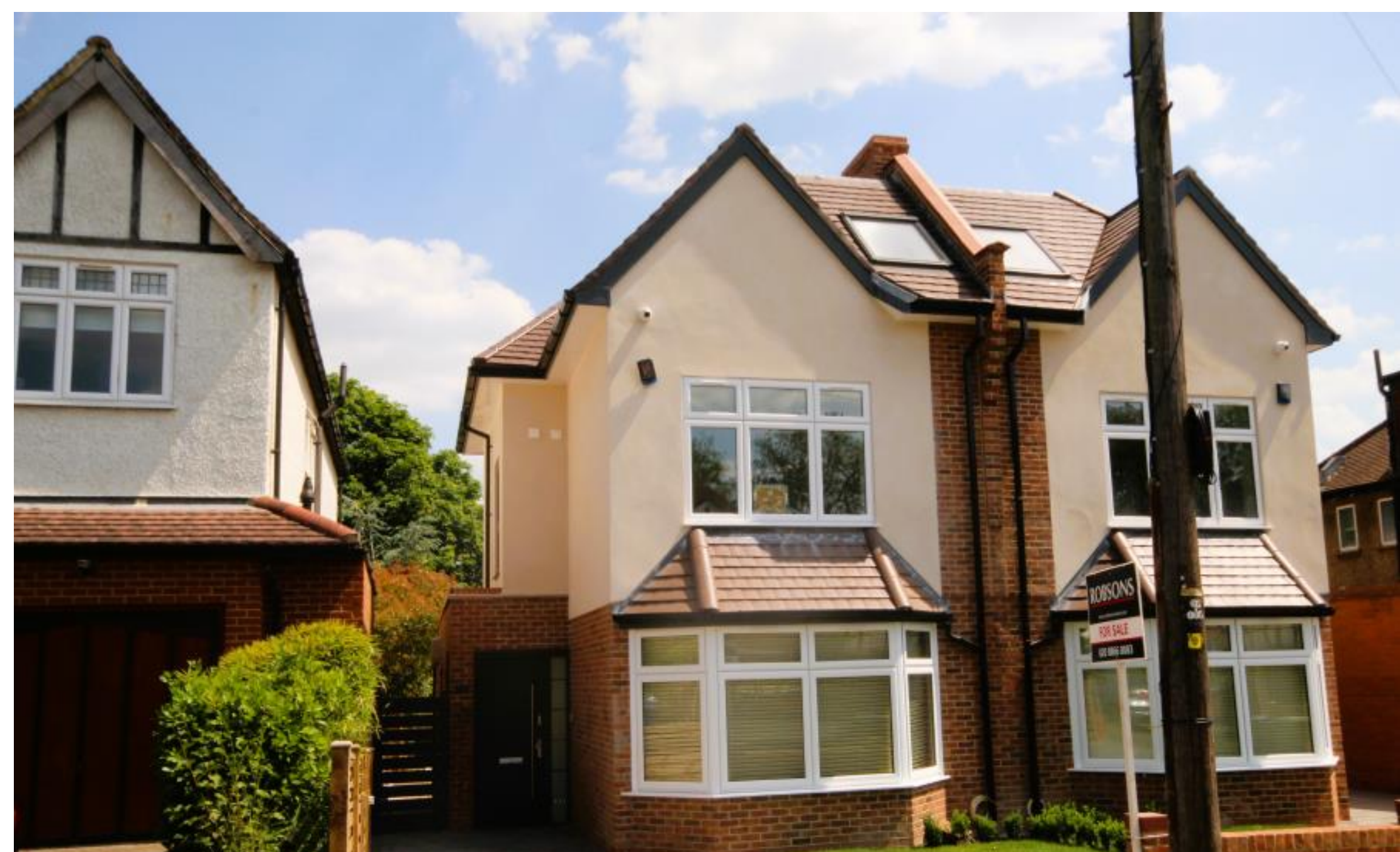
A brand new four bedroom, four bathroom family home in a sought after road Hillview Road, Pinner, Middlesex HA5 4PB
