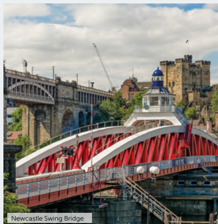
Newcastle Swing Bridge
