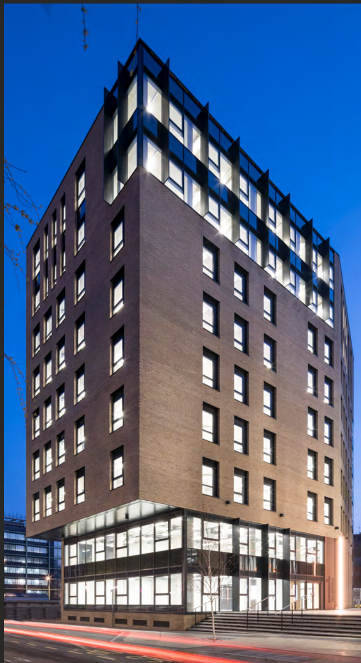
Exterior from Avon Street, entrance and reception
