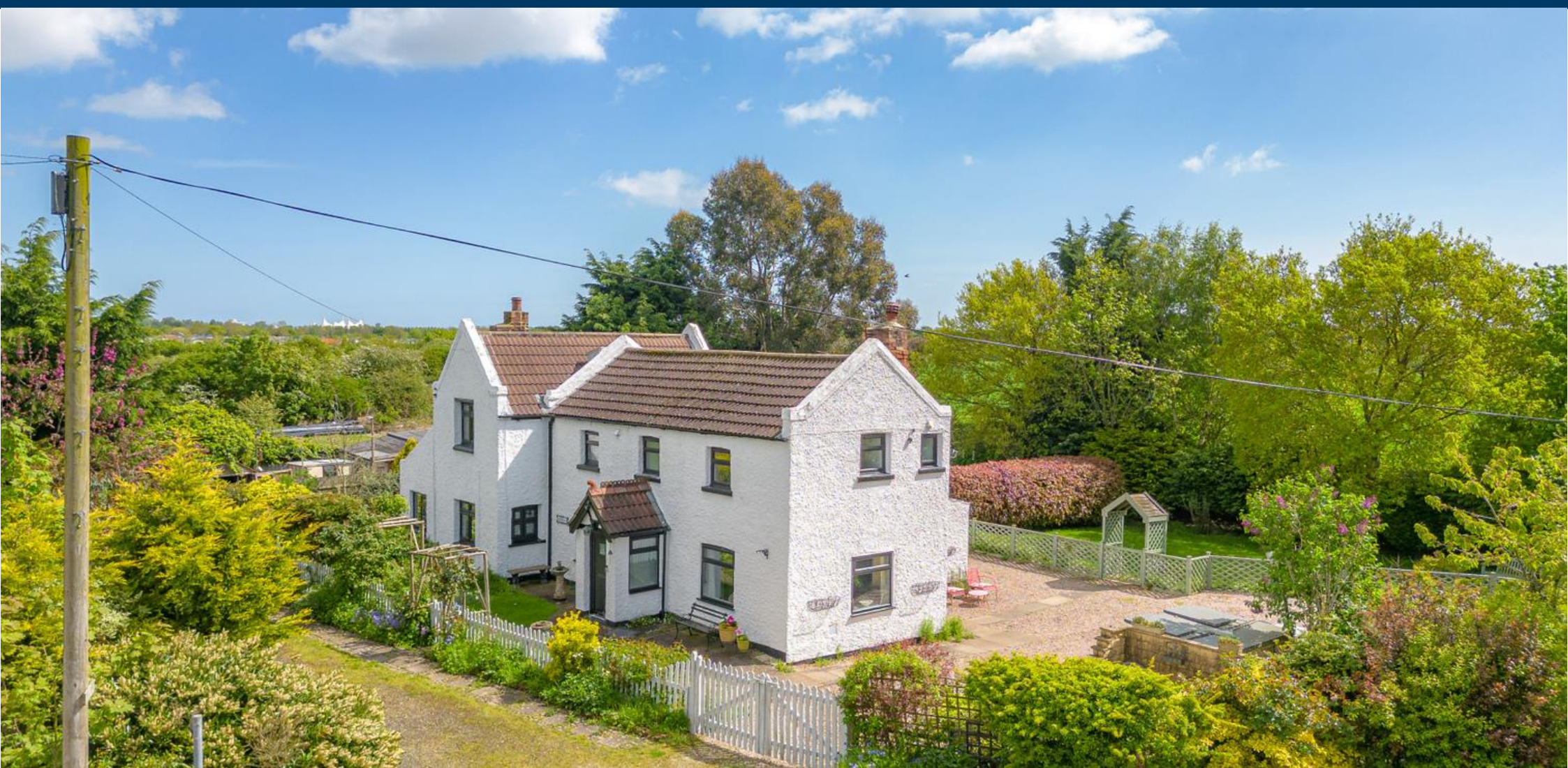
Pendle Cottage, Church End, Winthorpe, Skegness, PE25 1EJ
