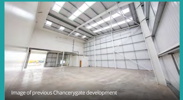
Image of previous Chancerygate development
