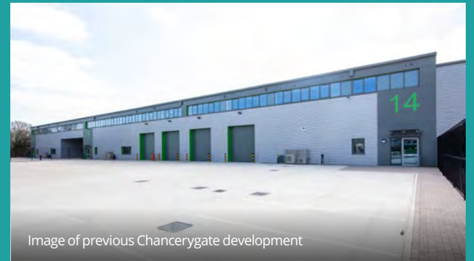
Image of previous Chancerygate development
