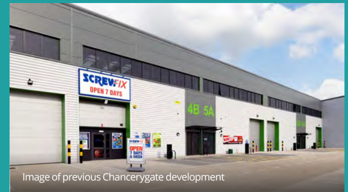
Image of previous Chancerygate development
