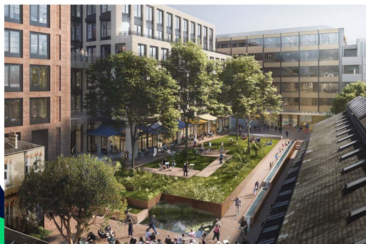
Dock Office Courtyard Practical Completion Q1 2025.
