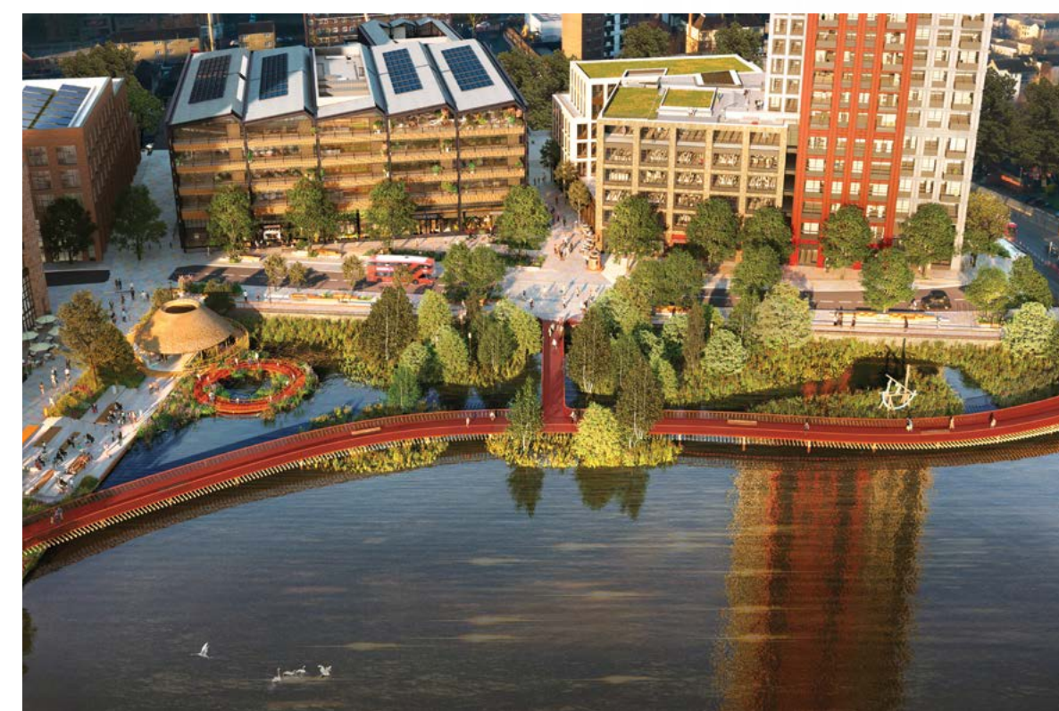
Canada Dock Phase 1 public realm. Practical Completion early 2024.
