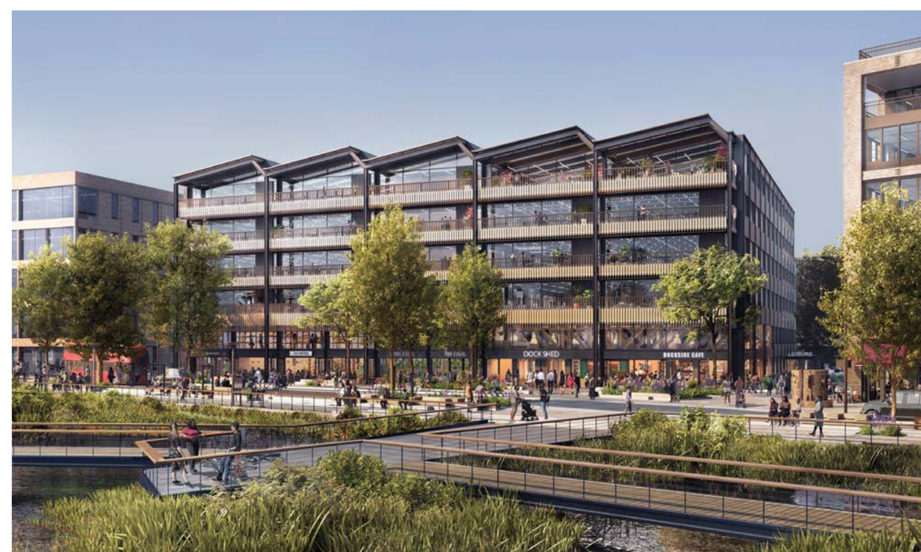
Dock Shed 180,941 sq ft. Practical Completion Q4 2024.
