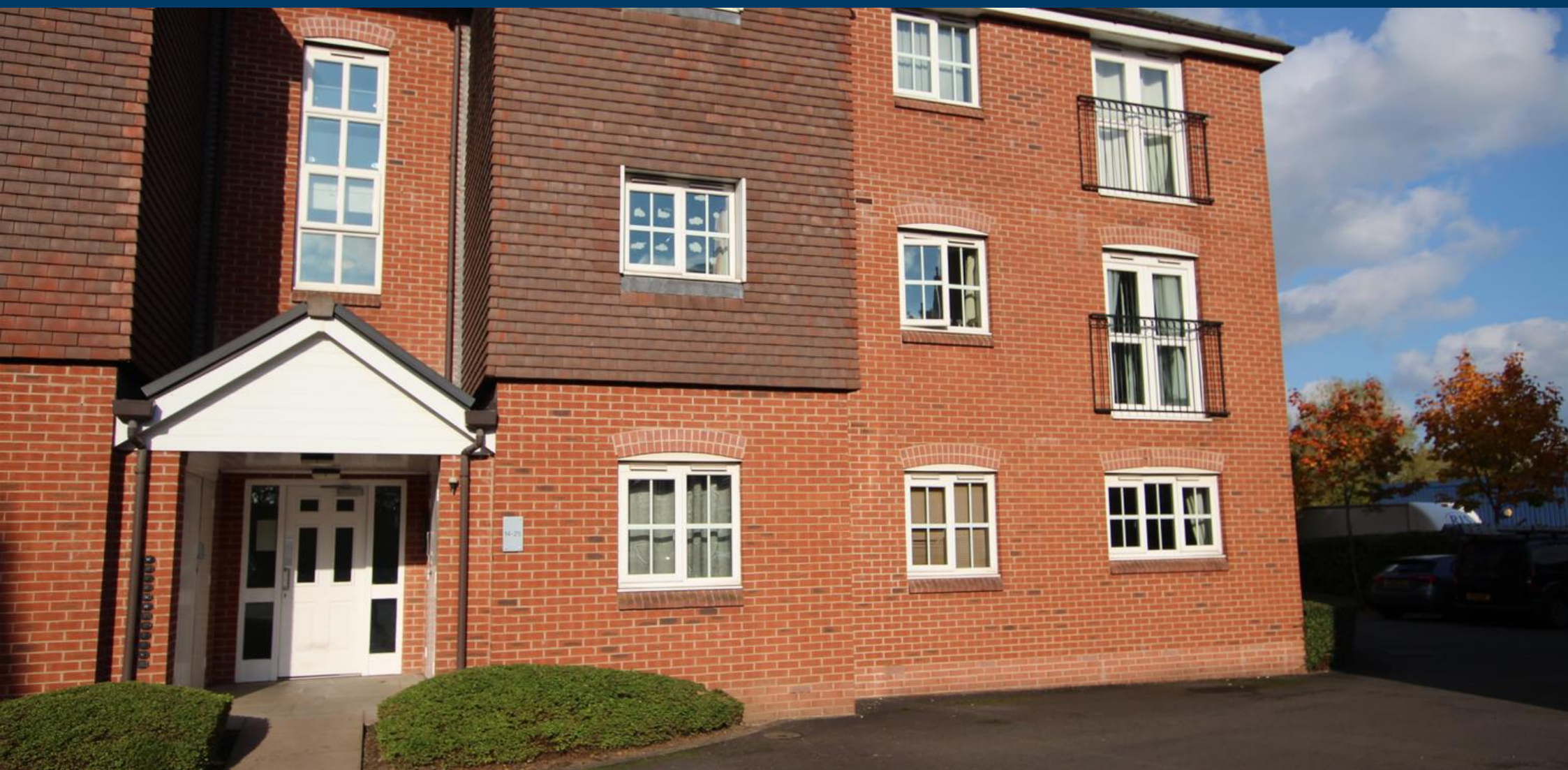
Hendeley Court, Burton-on-Trent
