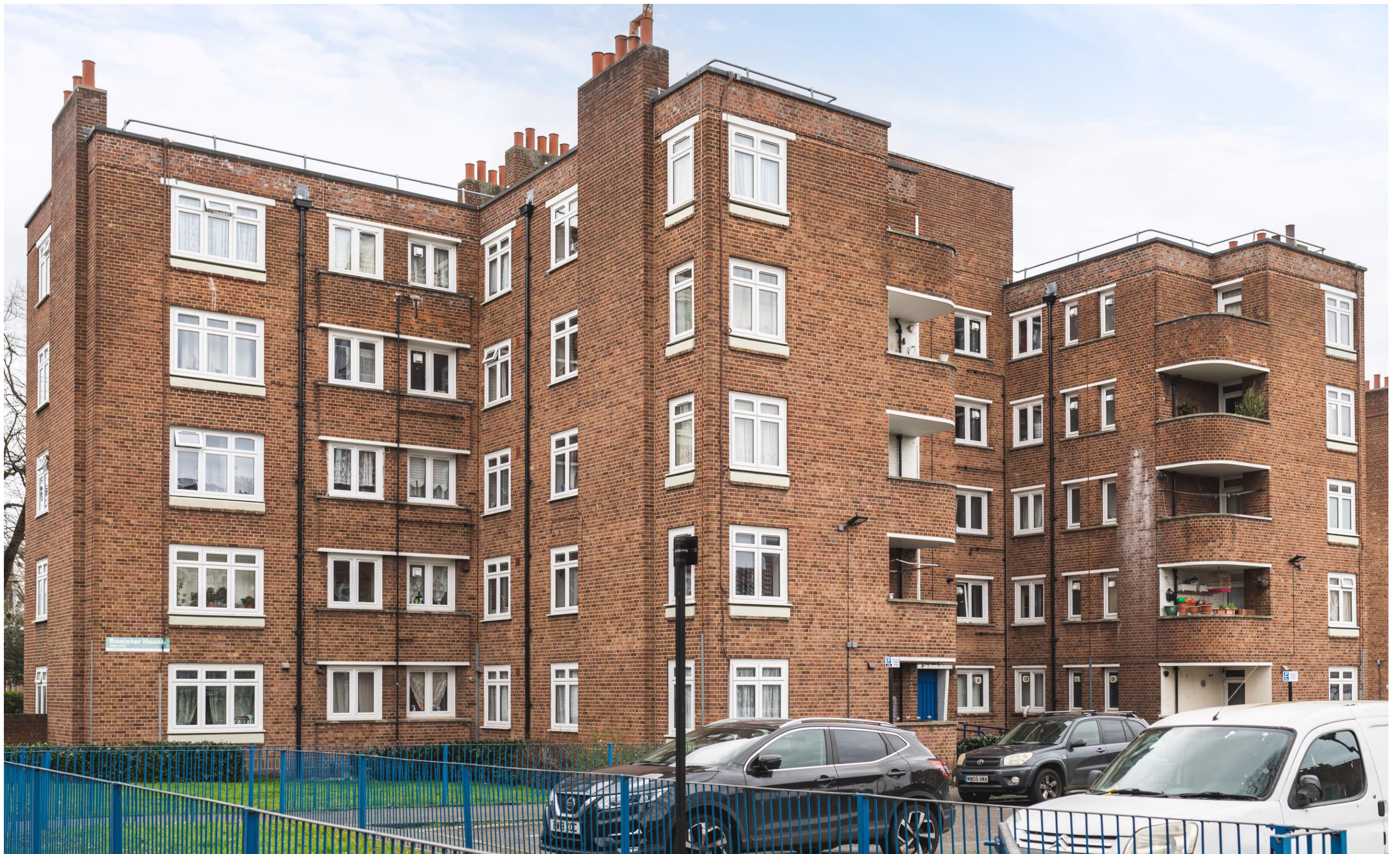
Banister House, Homerton High Street, E9 6BT
