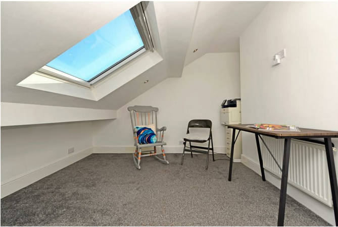
Velux window, central heating radiator
