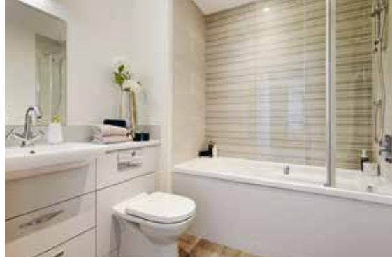
Ceramic wall tiling in bathrooms and en-suites
