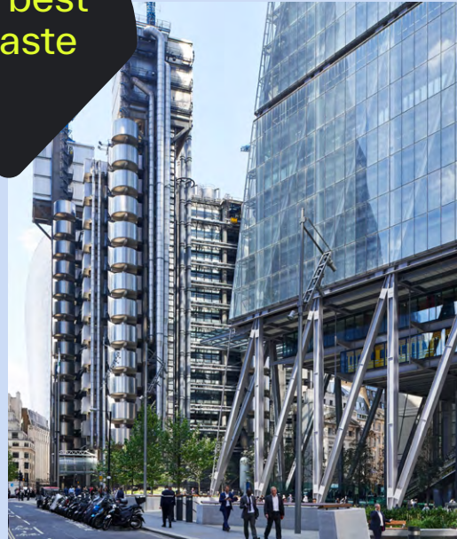
The Lloyds Building and The Leadenhall Building
