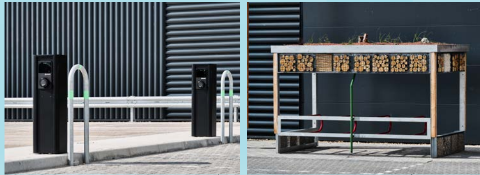
GREEN ROOF CYCLE SHELTERS
