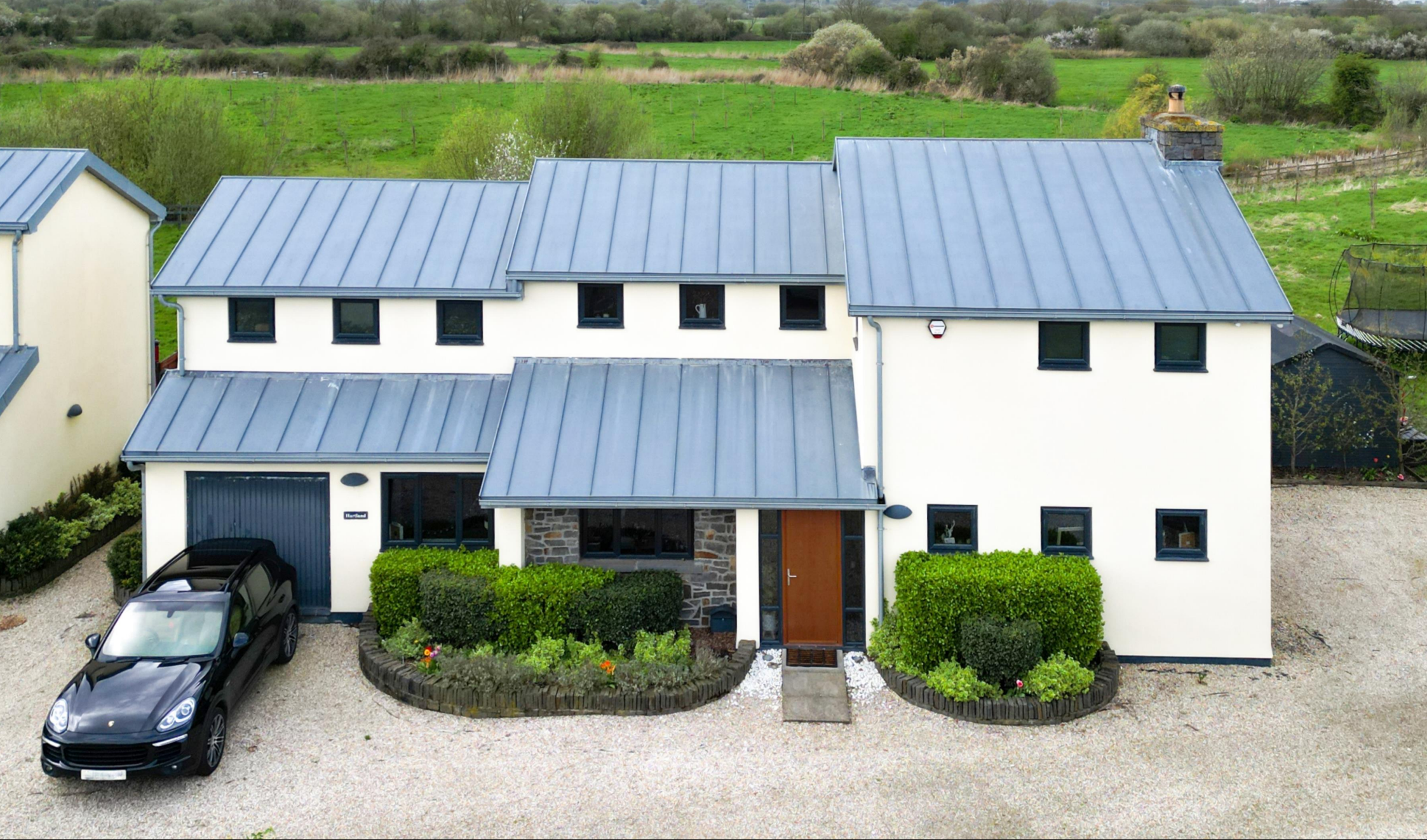
Hartland Cottage Church Road | St Brides | Newport | NP10 8SQ
