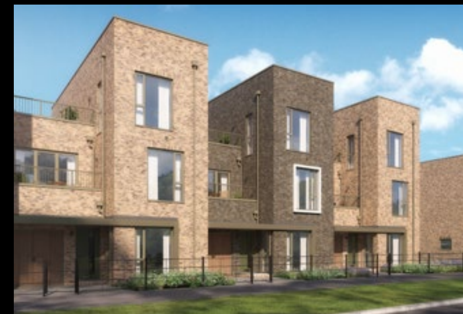
The De Havilland 4 bedroom mid and end terrace house with carport
