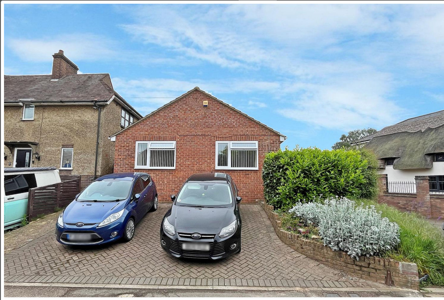
Hornes End Road, Flitwick, Bedfordshire MK45 1JH
