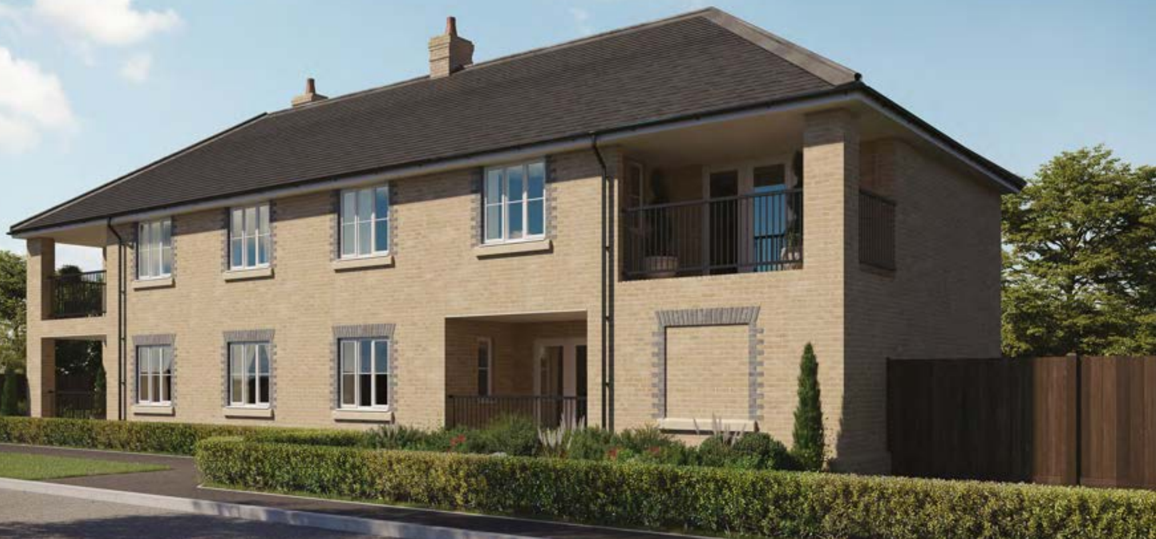
The Walsham Apartments
