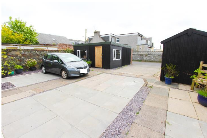
WORKSHOP: A large wooden workshop to the rear with service door and uPVC windows.
