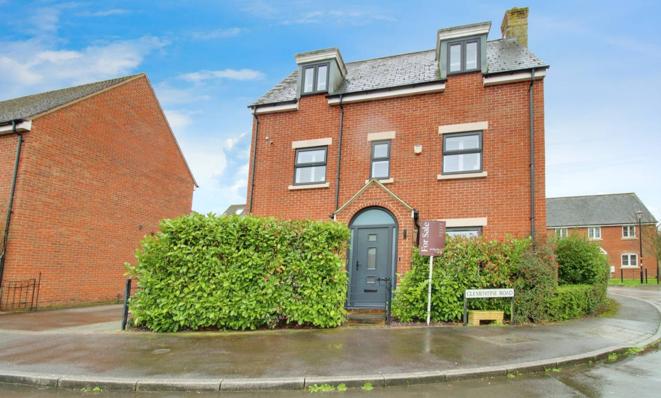
19 Clementine Road, Swindon Swindon
