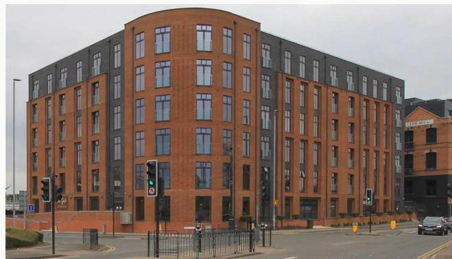
The Gate Waterside Village
