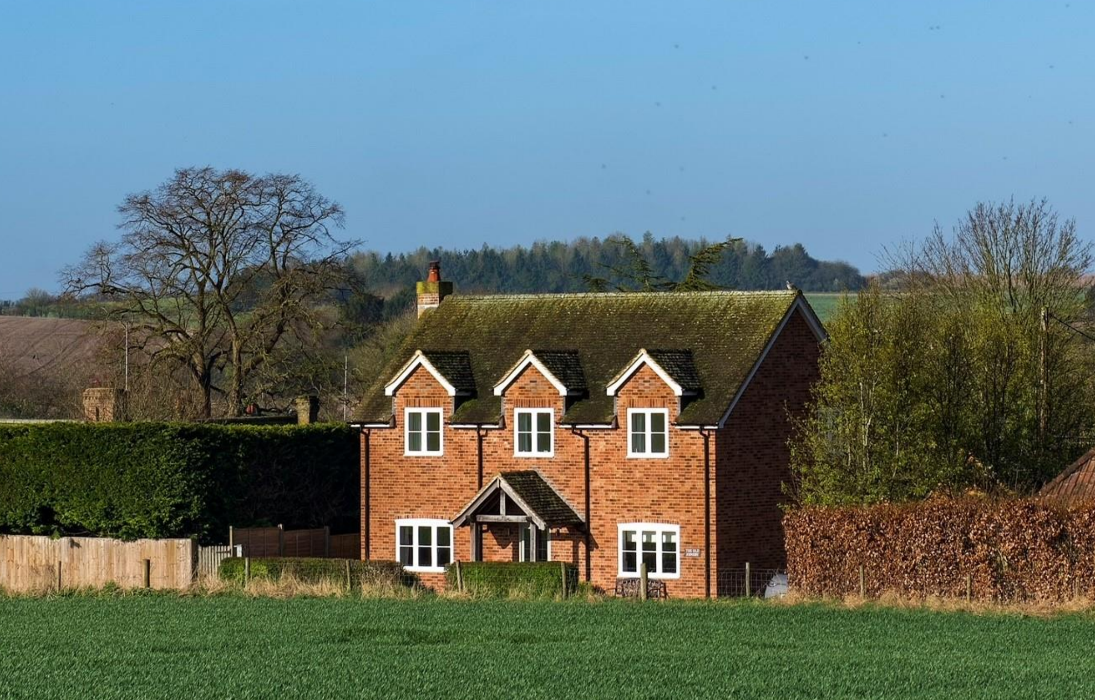
The Old Joinery, Barton Stacey
