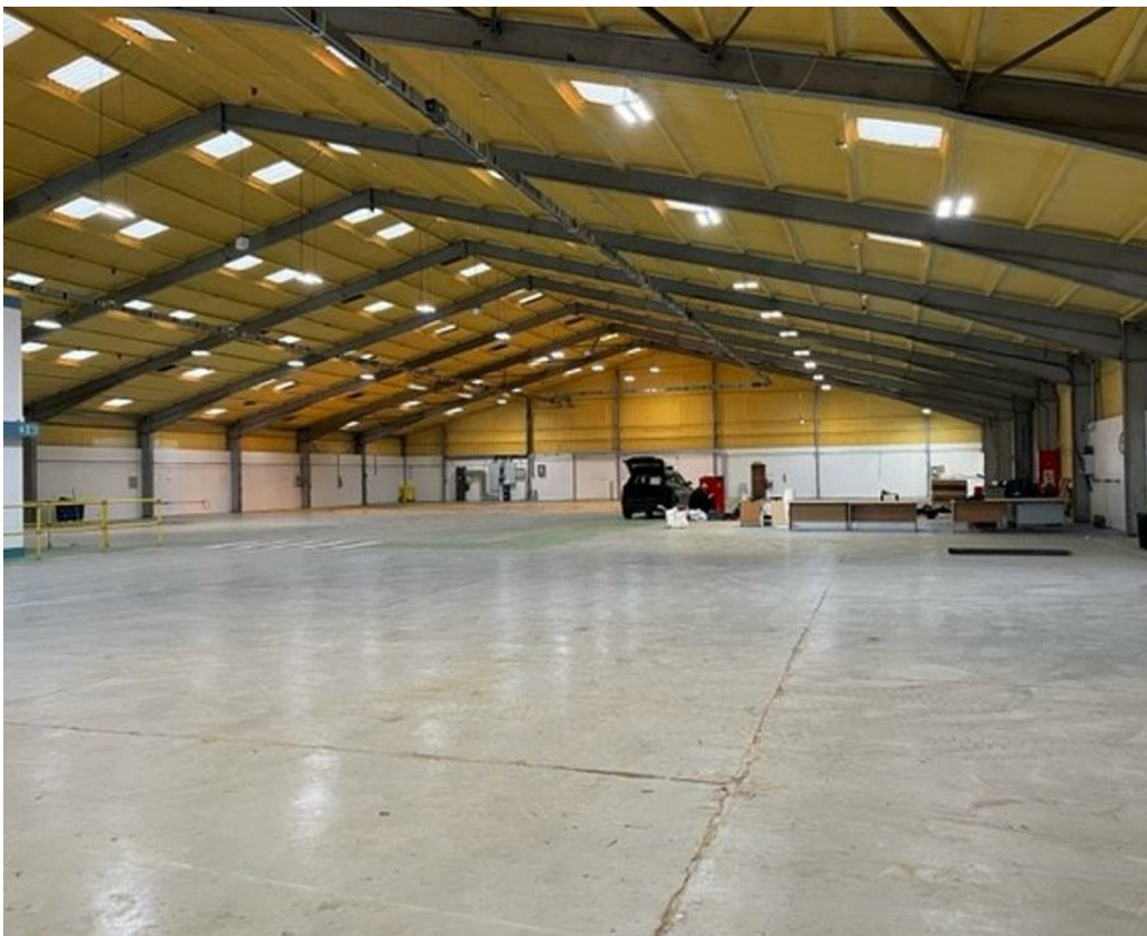
Internal views of the warehouse / production area
