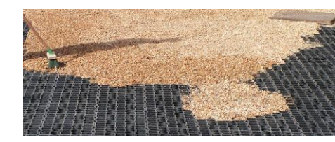
Stabilised Gravel Driveway
