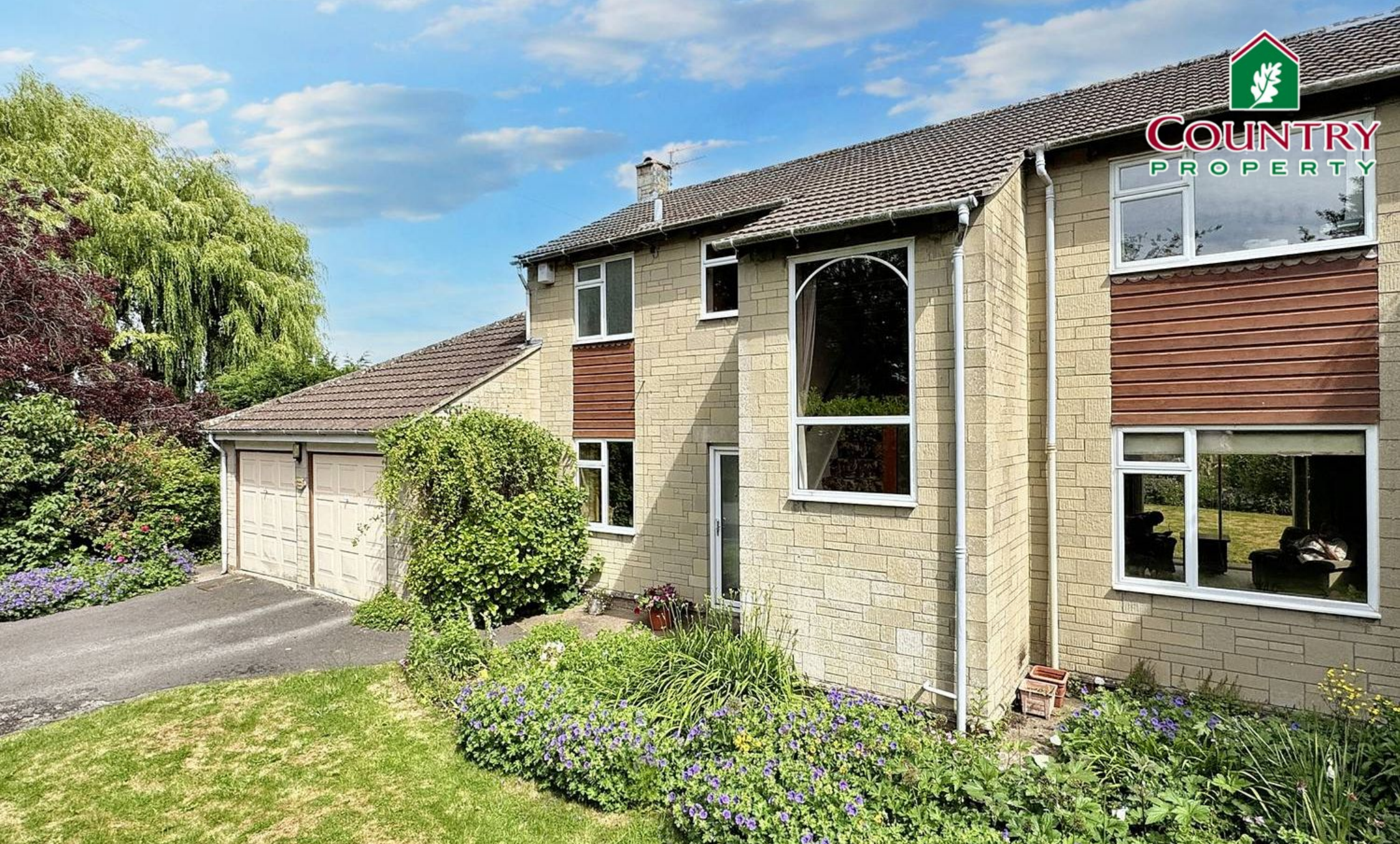
Becket House Pucklechurch
