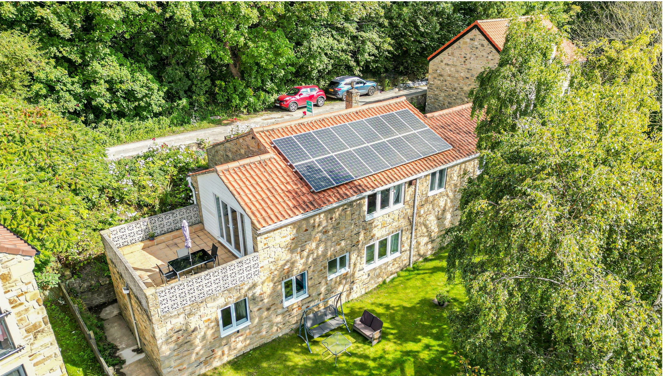
Carfu, Beckfield Lane, Fairburn, Knottingley, WF11 9JP £495,000
