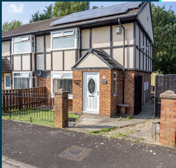
Bruntons Manor Court, Middlesbrough, TS3
