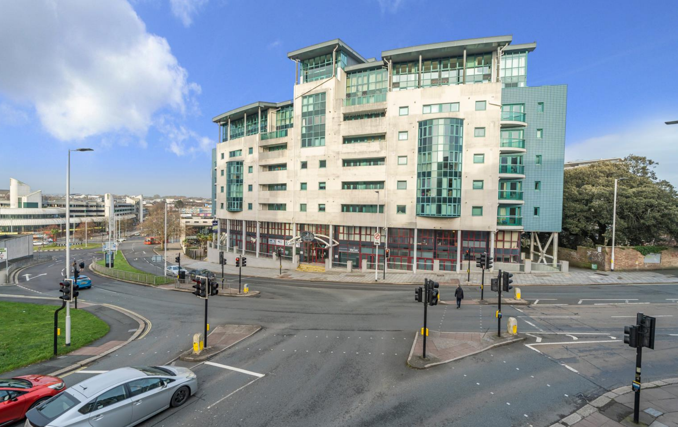
The Crescent , City Centre, Plymouth
