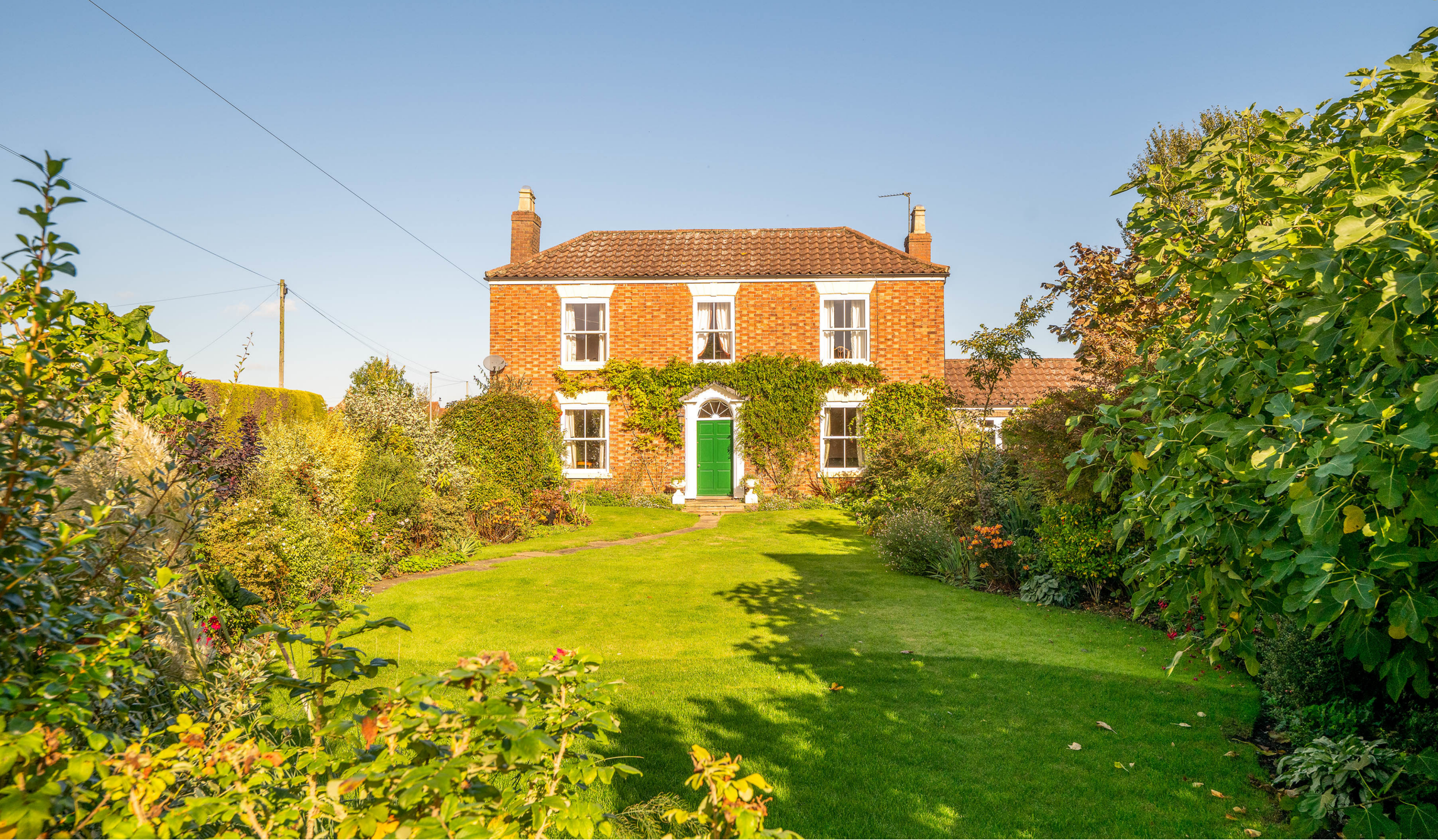
Bleak Farm House Misterton, Doncaster, South Yorkshire
