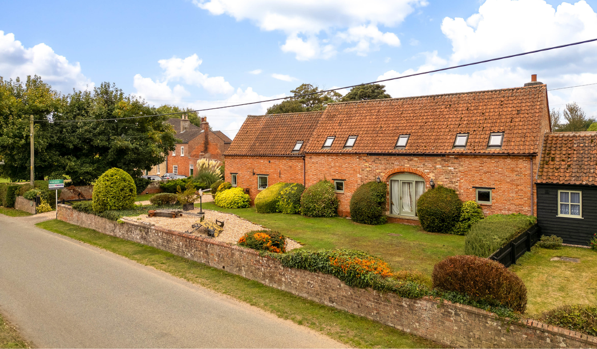
East Grange Barn Sleaford, Lincolnshire
